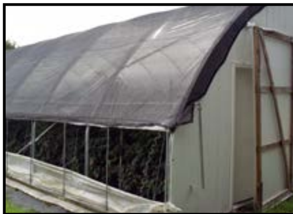
40% shade cloth installed on a high tunnel
