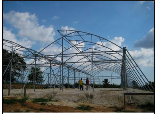
Structure under construction using a metal frame in Middlesex
