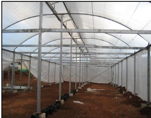
Note cross-bracing on the end-walls of this metal frame structure
