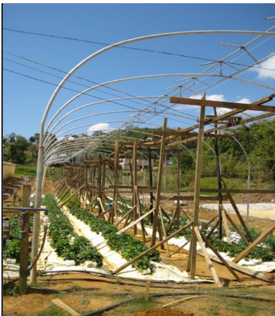
Structure in Christiana constructed with wood frame and metal ribs
