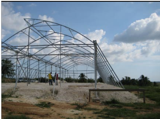
Metal-frame structure being constructed on elevated pad
