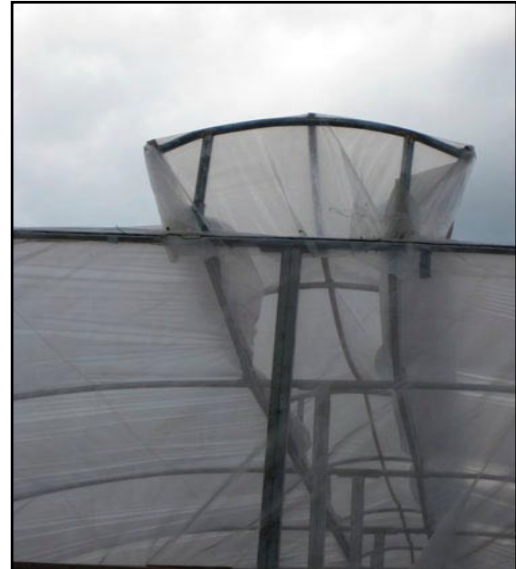
Anti-viral screen covering a double ridge vent.
