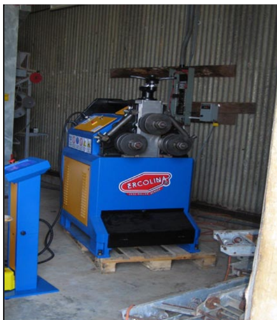
Pipe bender used to manufacture metal ribs in Christiana
